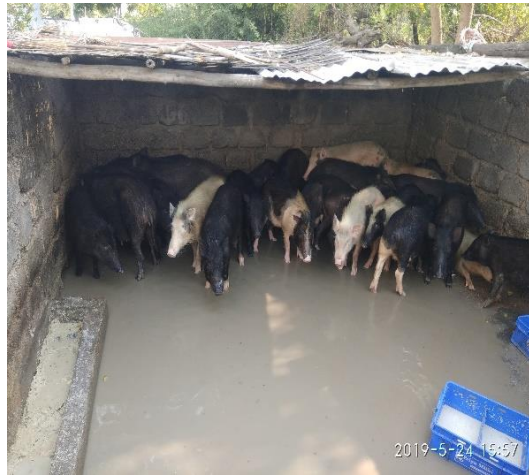
Fig 13: Pig sty with inefficient drainage
