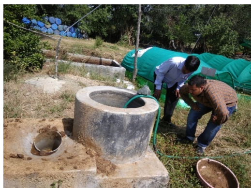
Water feeding in inlet of biogas plant
