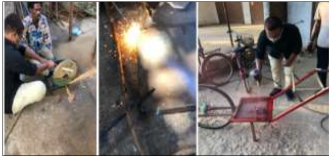
Fig 6: Construction assembly of main frame
