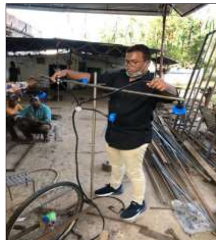
Fig 9: installations of nozzle & pipe
