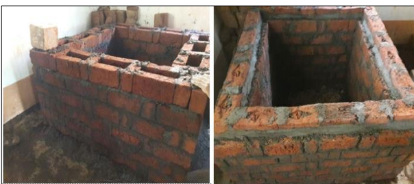
Plate 1: Construction Rat Trap Bond Masonary Onion Storage Structure
