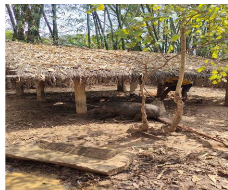
Temporary shelter (Wooden Housing roof with longleaf Indian pine)
