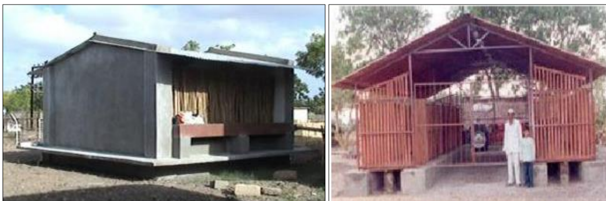
Plate 9: Forced air ventilated storage structure
