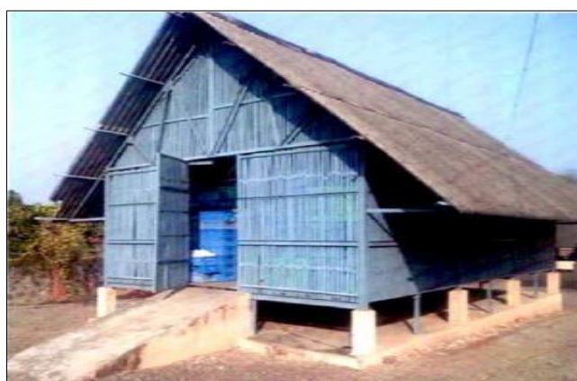
Plate 13: Top and bottom ventilated storage structure with mud plastered walls
