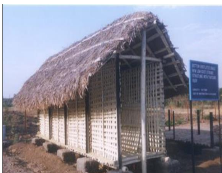
Plate 17: Low-cost bottom ventilated onion storage structure
