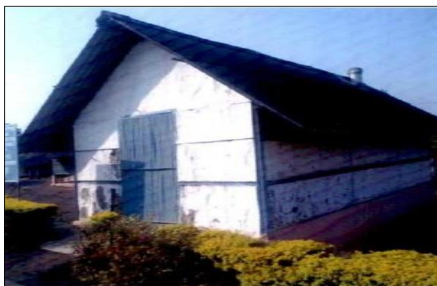
Plate 12: Modified Bottom ventilated storage structure chain linked side walls
