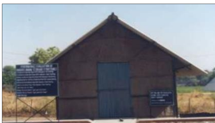
Plate 10: Top and bottom ventilated storage structure with mud-plastered walls
