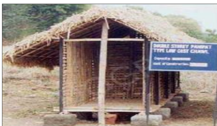
Plate 11: Bottom ventilated single row low-cost thatched roof storage structure
